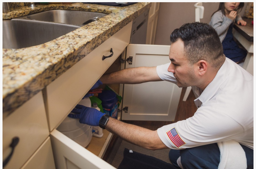
gilbert plumber leak repair
