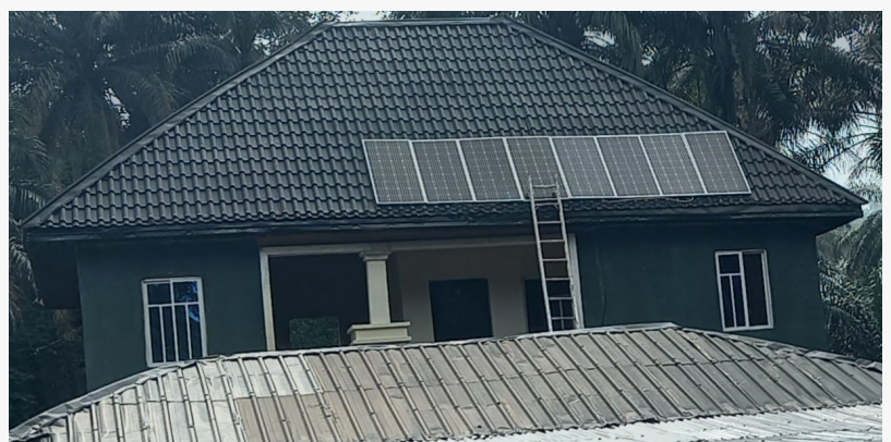
JMeggro is powered by a 5KVA solar system
