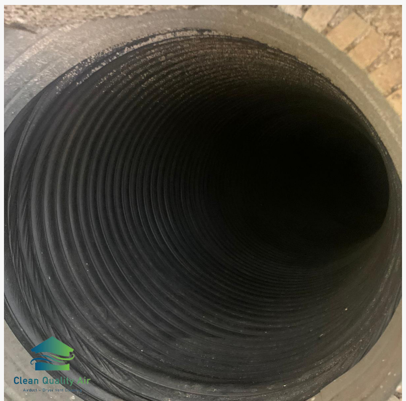
Air Duct Cleaning Port St Lucie
