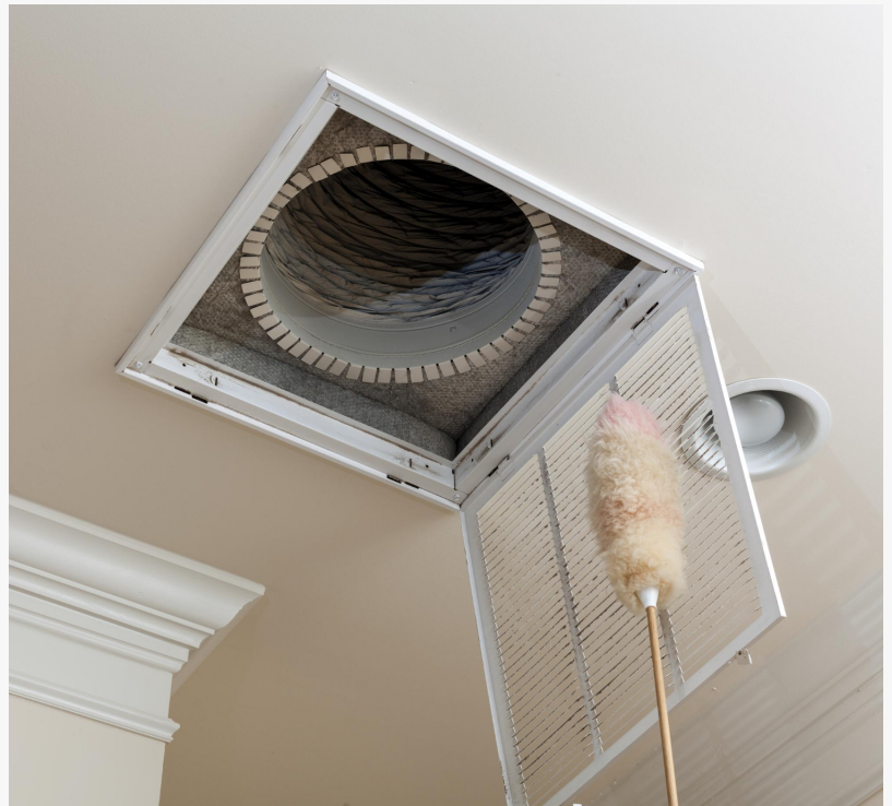
Air Duct Cleaning PSL
