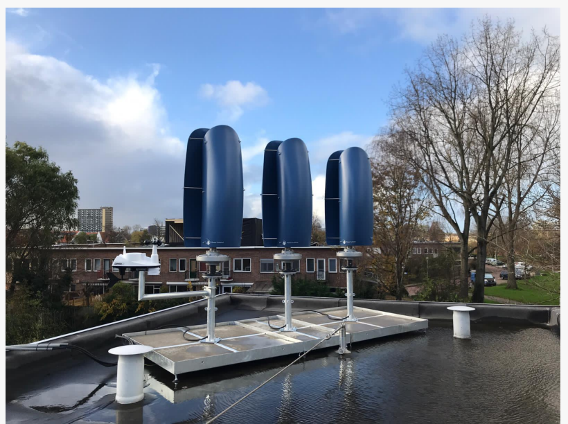
Three installed small size Wind Tulips
