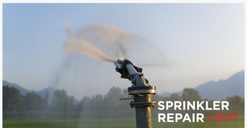
Irrigation Sprinkler Repair in Dallas
