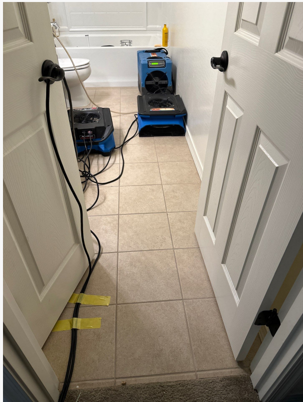
Water Damage equipment set up to dry out this bathroom.
