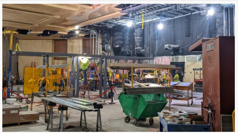
Expansion work inside the Hollywood Casino Toledo.
