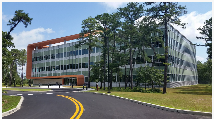
The fully occupied first of seven planned multi-story buildings that will comprise the National Aerospace Research & Technology Park (NARTP) in Atlantic County, NJ.
