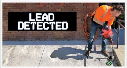
Using Electro Scan's SWORDFISH buried lead pipe can be confirmed from accessing curbstop locations or from inside buildings at the meter.
