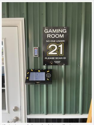
ID Activated door lock installation on the gaming room at an Illinois grocery store
