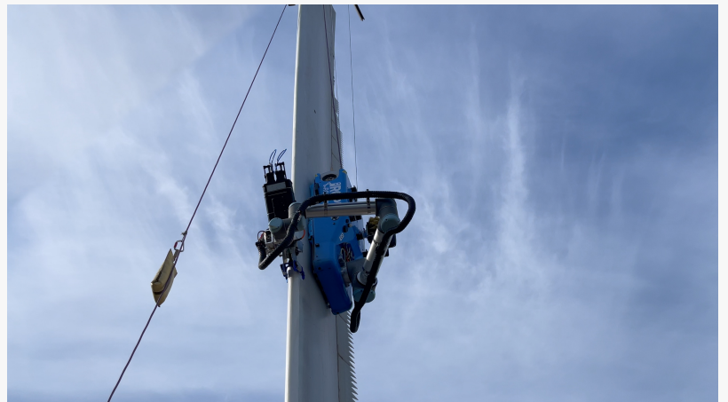
The robot applies viscous material to rebuild the leading-edge of the blade. The patented spreader tool smooths the surface to create an optimal aerodynamic edge.
