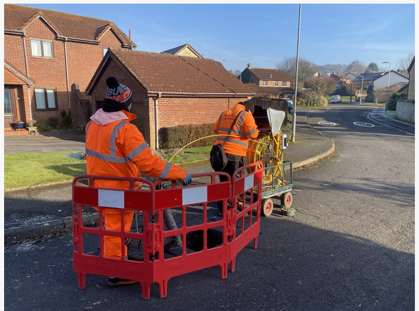
Electro Scan's British field team scan sewers to locate leak locations and severities to prioritise repairs and rehabilitation to prevent sewer backups and flooding.
