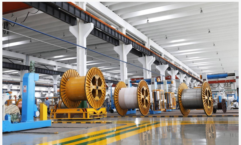
Electric Cable Plant
