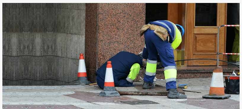
Drain Repairs ASAP Drainage
