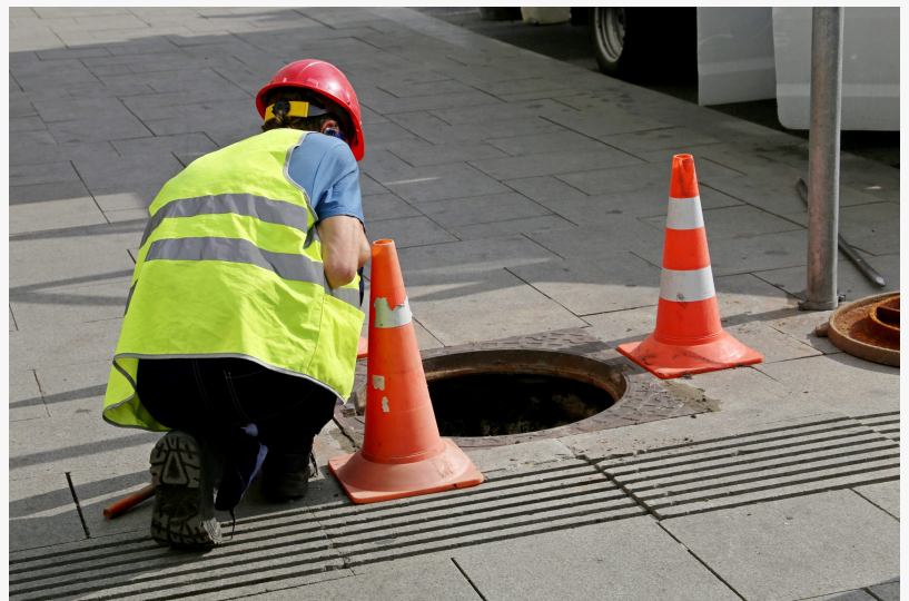
Drain Lining ASAP Drainage
