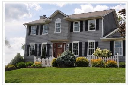
Builders and remodelers can use insulated vinyl siding to help meet the energy code's continuous insulation requirements. Insulated vinyl siding is engineered to incorporate a substantial insulation thickness of at least R-2.
