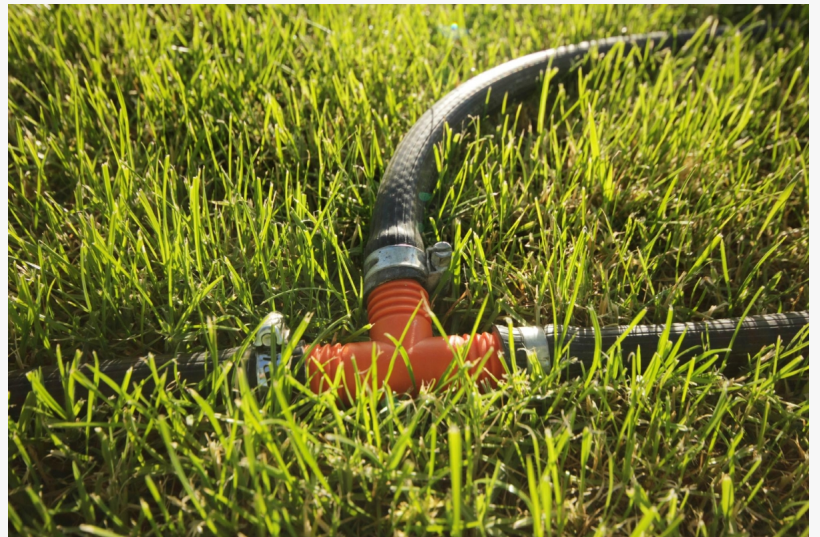
Drainage Installation in Irving, Texas
