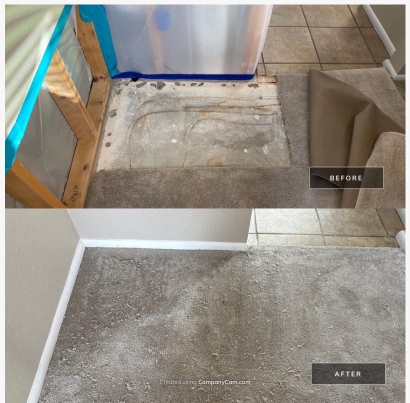
Carpet repair after water damage restoration was complete.
