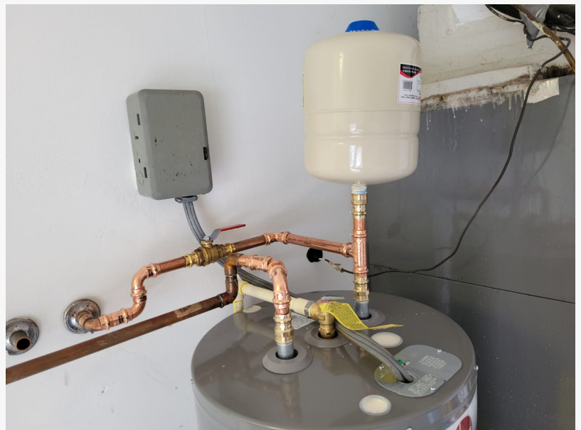
The Water Heater Heroes LLC
