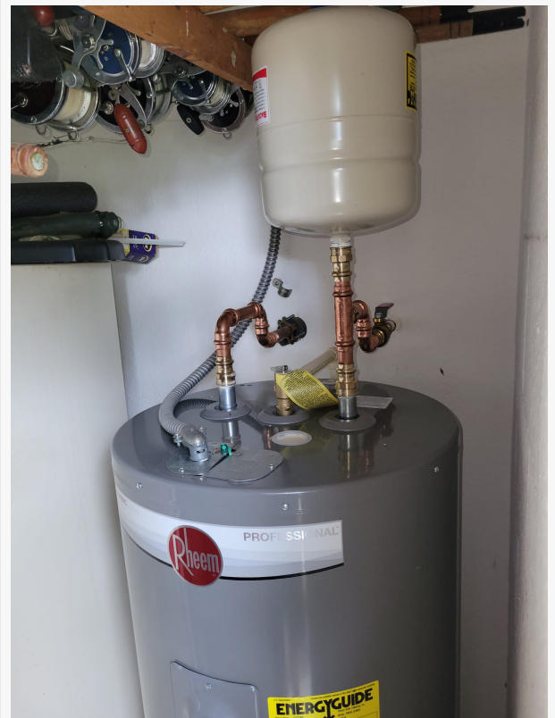
Water Heater Repair
