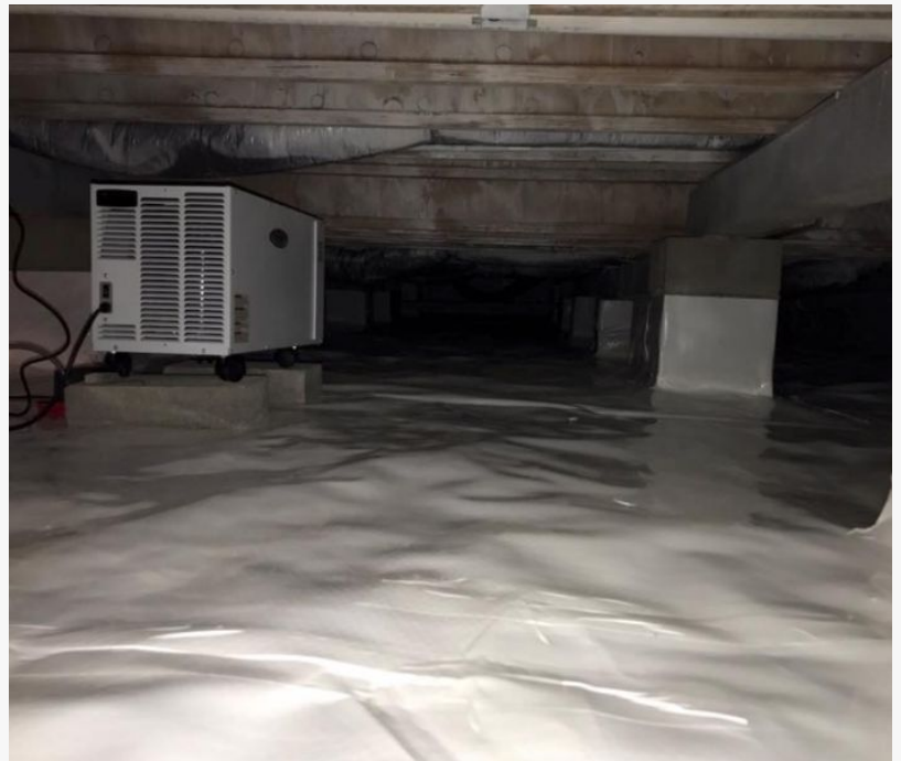
after crawl space vapor barrier and dehumidifier installation for a home
