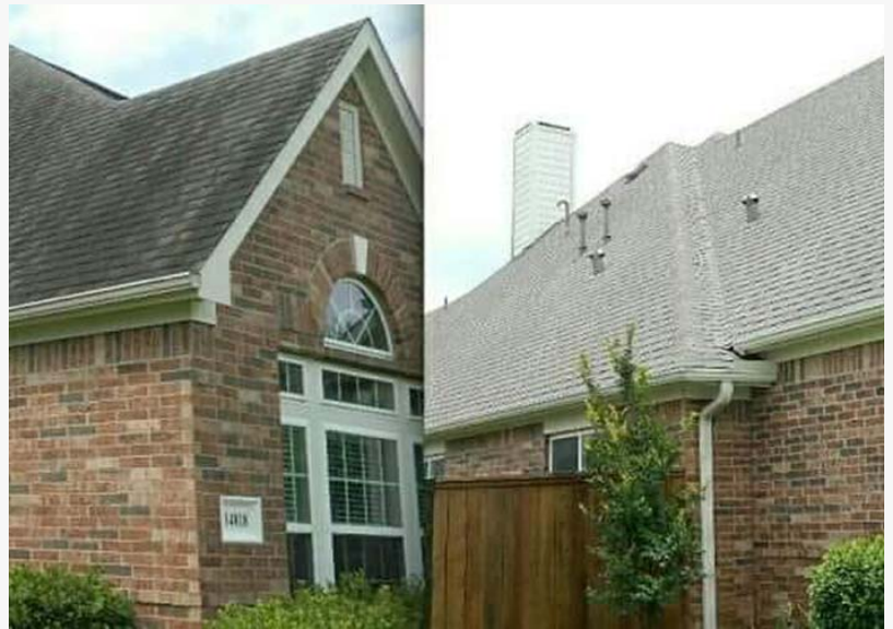
before and after power washing a shingle roof
