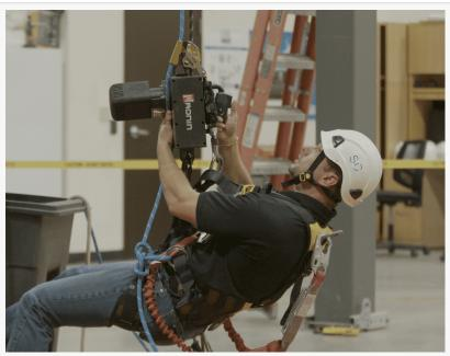
The Ronin Lift evolved from elite military technology that enables SAC Wireless technicians to ascend quickly and safely to elevated work locations.
