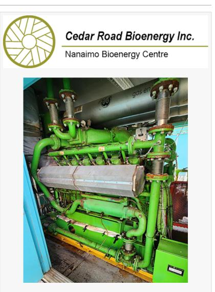
housed in a 40" sea container; including spare parts; Gas Booster, Gas Conditioning Skid, and Dehydration Unit; Tecon 1266 Cu/M biogas storage Unit; Distribution Substations (25 KVA High voltage cabinet with 1 MW transformer steeped down to lower volage genset breaker cabinet; and various storage containers.
