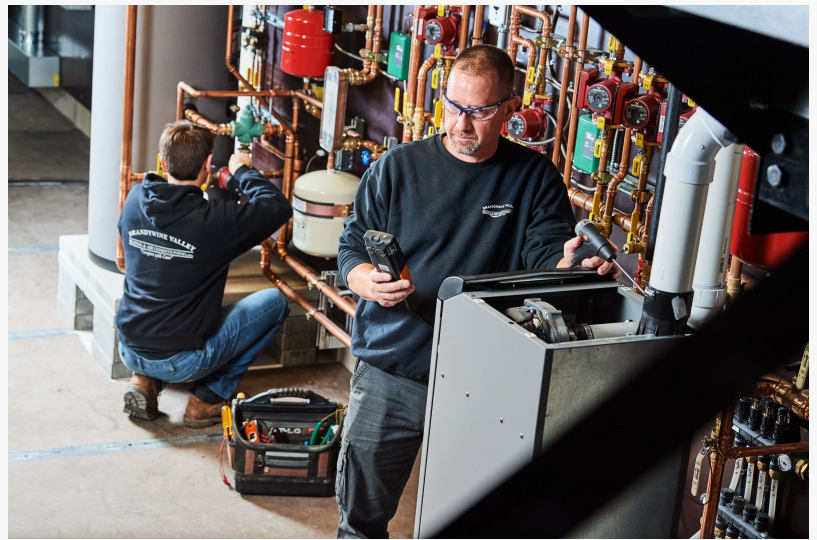
Brandywine Valley HVAC Techs at work
