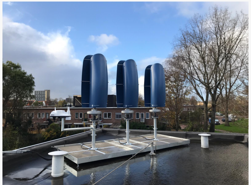
Three installed small size Wind Tulips
