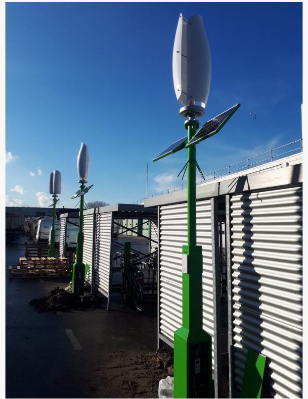
Wind and Solar E-bike Charging Poles
