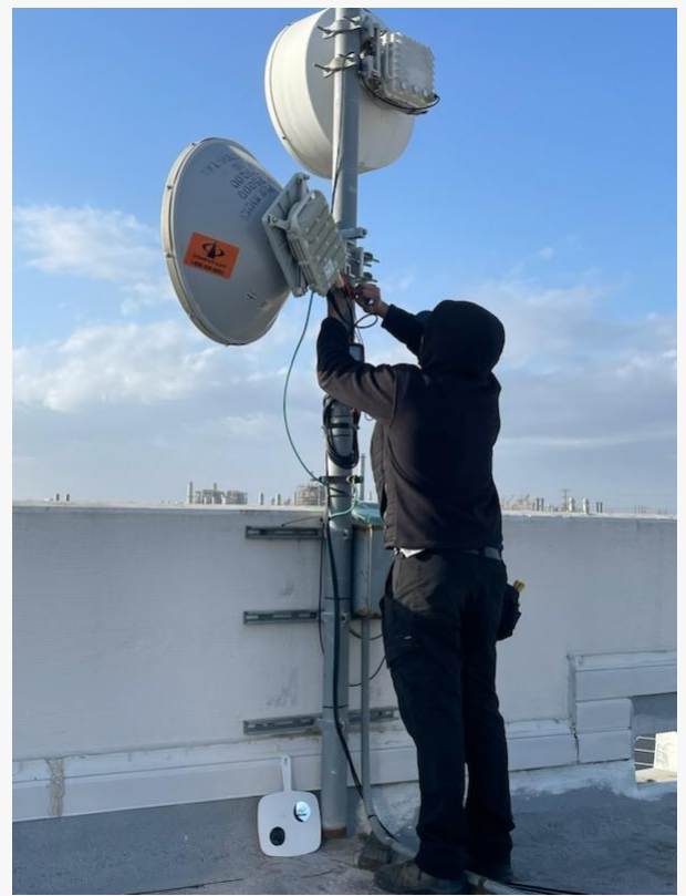
Towerstream engineer works on fixed wireless radio to install 10Gbps connection.
