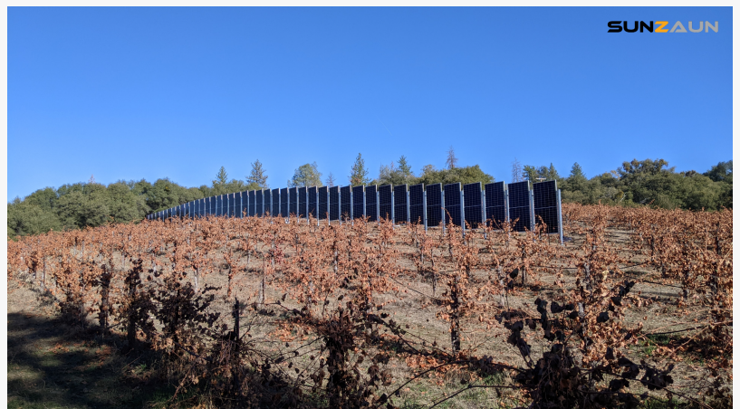
The vertical orientation of the panels is ideal for agrivoltaic applications
