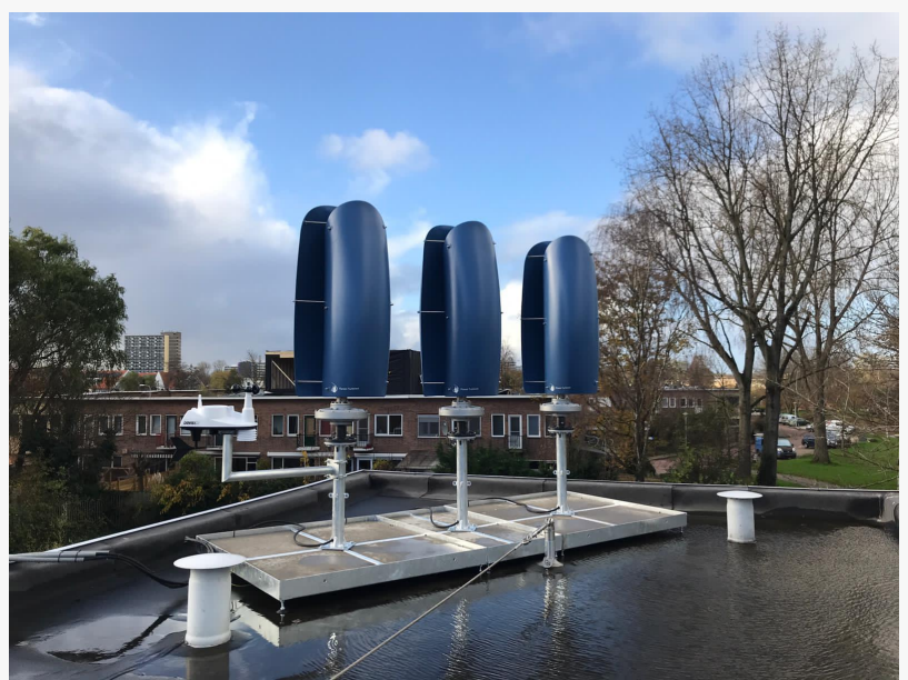
Three installed small size Wind Tulips
