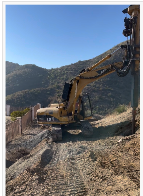
JVC ADU BUILDERS Construction Services
