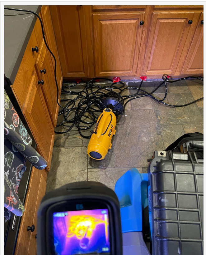
gilbert az water damage clean up
