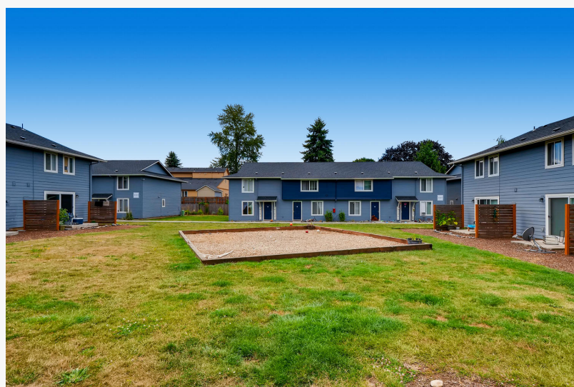
Wellington Court Exterior Green Space
