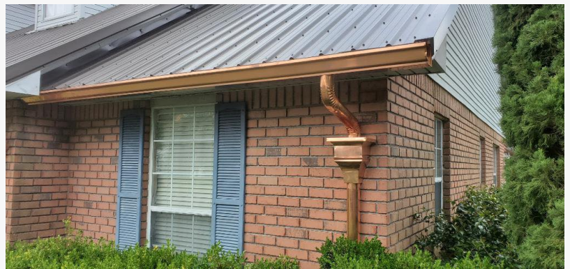
Pensacola Gutter Installation
