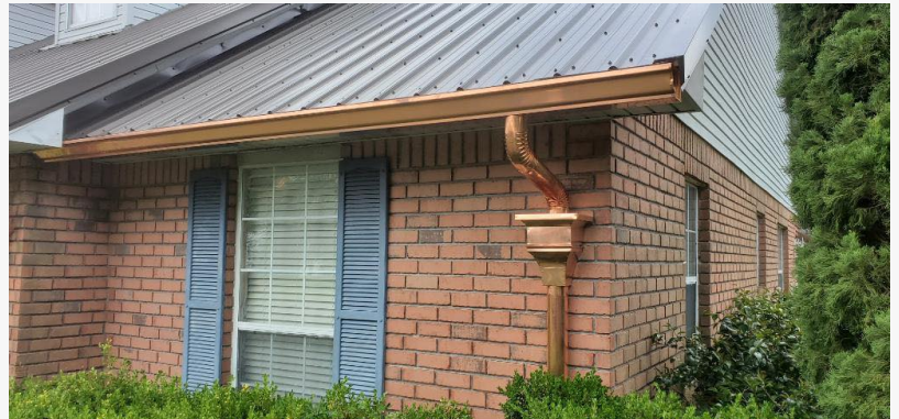
Pensacola Gutter Installation
