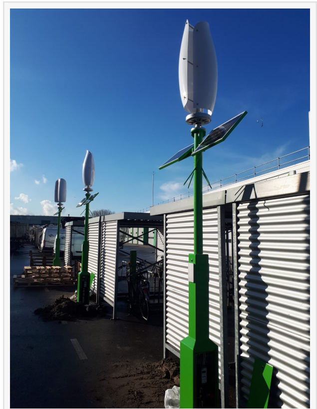
Wind and Solar E-bike Charging Poles
