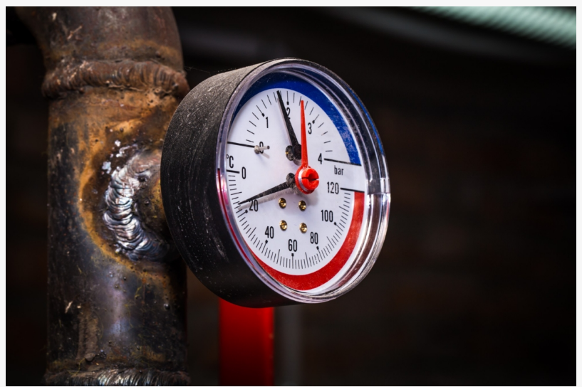
Leak Detection Service in Florida
