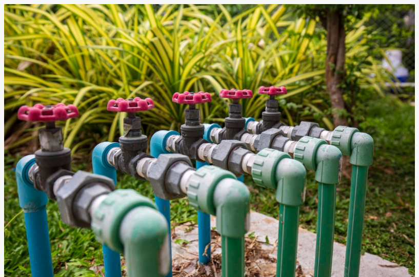
Plumbing Services Florida
