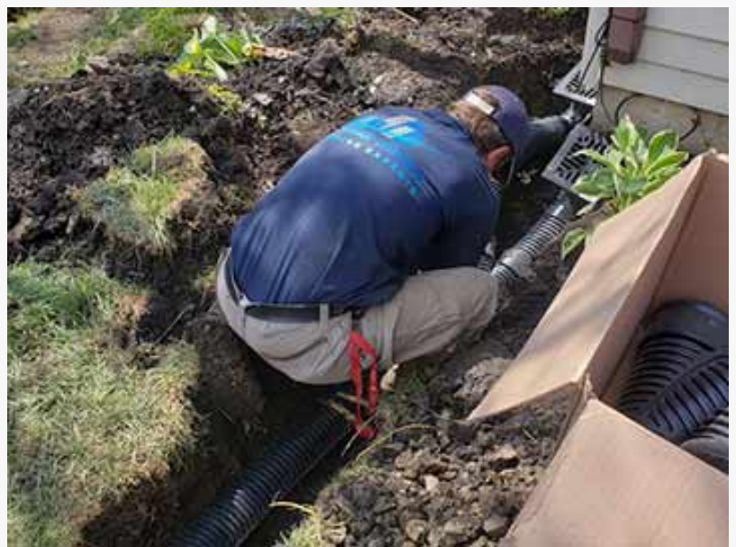
A French Drain Being Installed for a Customer in Brookfield, IL
