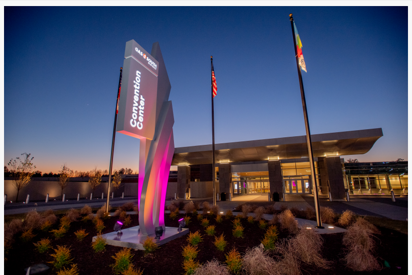
Gas South Convention Center
