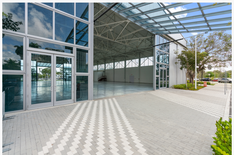
Grove Bay - Looking into a hangar through a raised bay door
