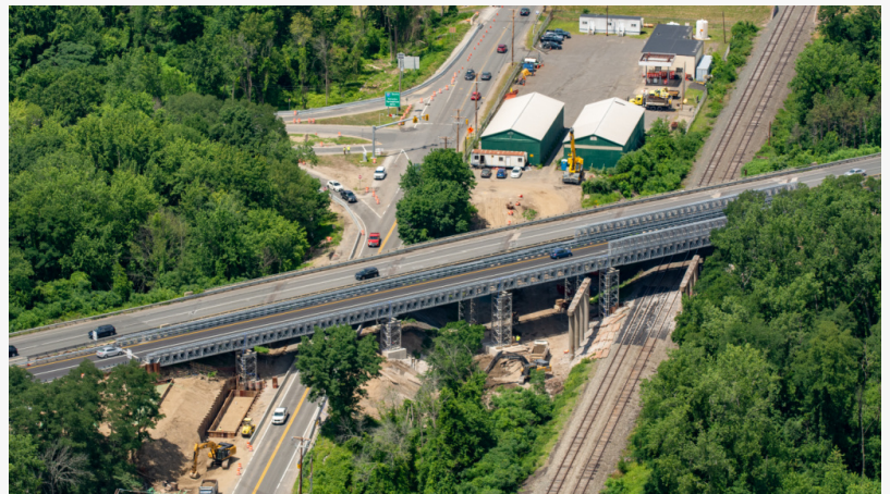
Acrow Temporary Bridge over U.S. Route 5 and B&M Railroad
