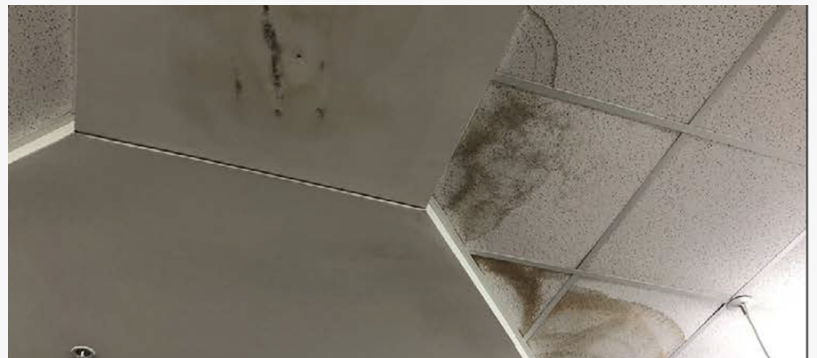
Here is a before photo of a School that needed Air testing and filters changed.
