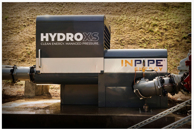
InPipe Energy HydroXS installed within footprint of water utility's existing pipeline infrastructure.
