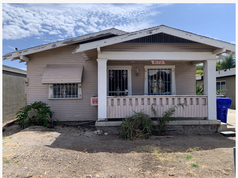
Buying Damaged Homes in San Diego
