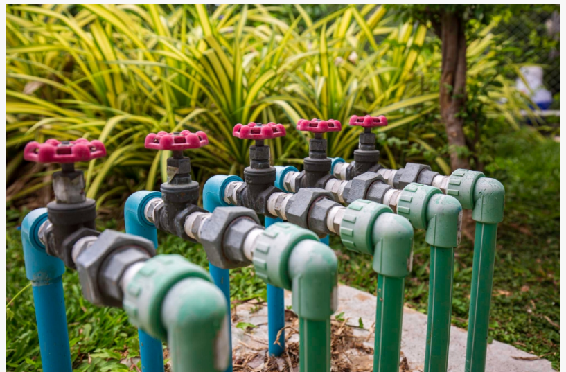
Pipe Surgeons - Professional Pipe Repair Services
