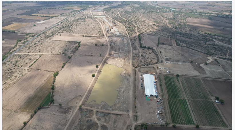
Construction of Check Dams by Dholakia Foundation
