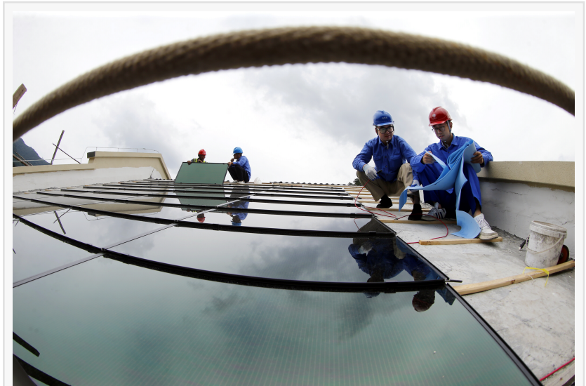
Roof installation of power generation glass
