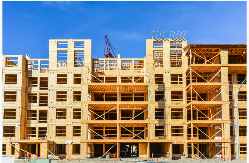
New multifamily development under construction
