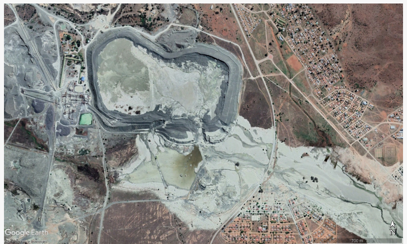
Post-failure satellite image of the Jagersfontein dam. Source: Google Earth Pro
