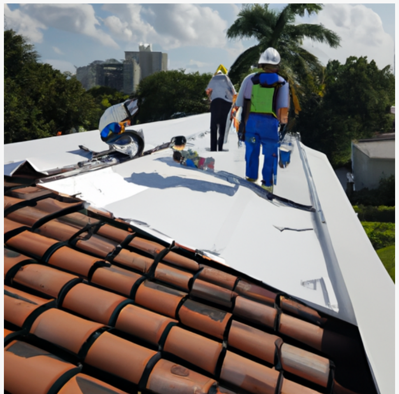
Roofers in Miami FL
