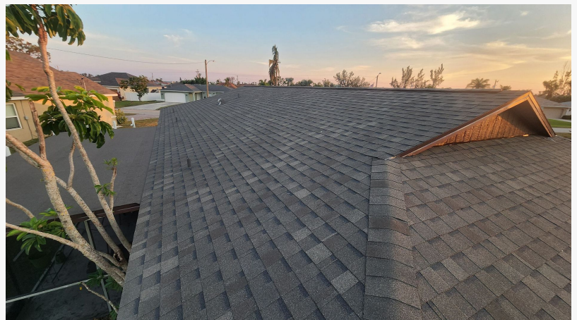
emergency roof leak repair
