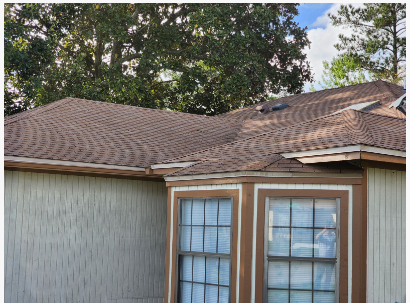
leaking roof repair in Jacksonville
