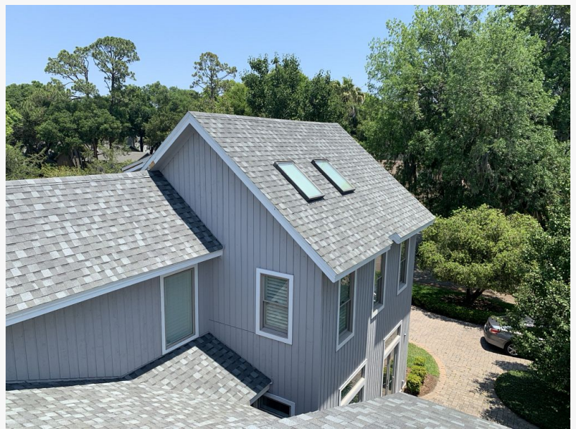
roof leak repair in Jacksonville
