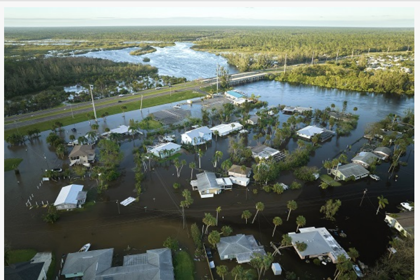
Hurricane Ian damage
