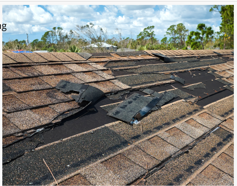
DAMAGED SHINGLES
